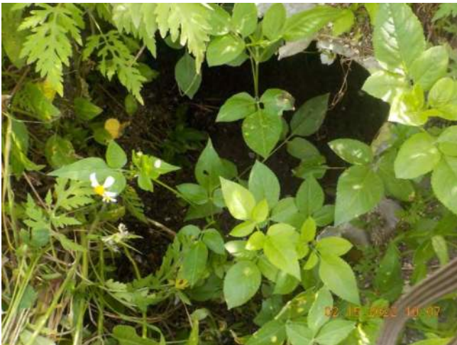
Photo 33: West side of the culvert leading to the LWDD E-2W.
