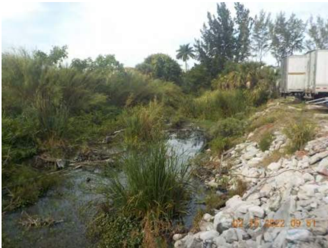
Photo 26: Point 2, standing water above ground (DSCN2914).
