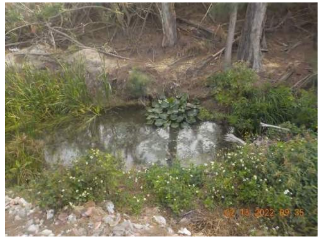
Photo 11: Point 1, overview of point with 8+ inches of standing water (DSCN2882).
