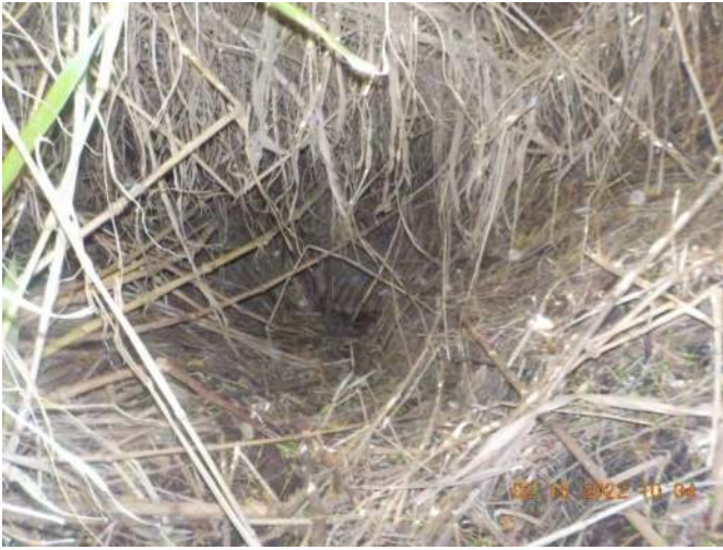
Photo 32: East side of the culvert leading to the LWDD E-2W.
