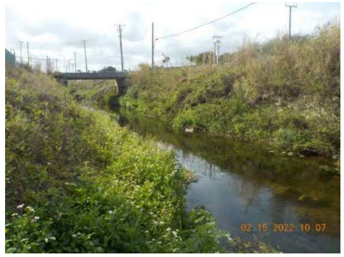
Photo 34: West side of property and the LWDD E-2W.
