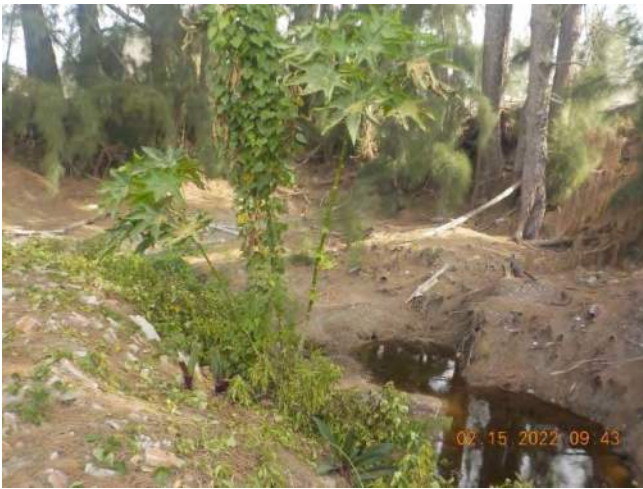
Photo 19: View North on NE corner of property, standing water in ditch.
