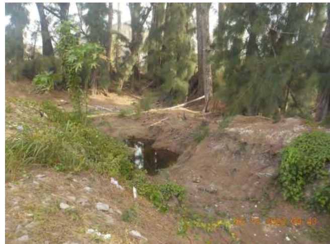
Photo 18: View North on NE corner of property, standing water in ditch.
