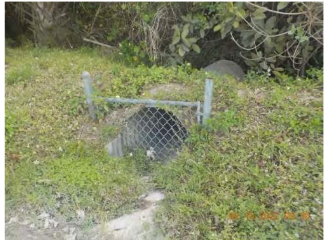
Photo 4: Culvert 30ft from southeast corner of the property.
