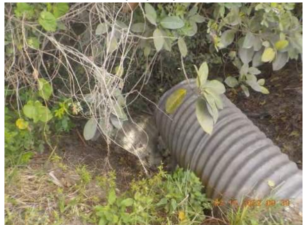
Photo 5: Culvert 30ft from southeast corner of the property.
