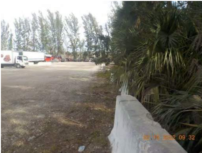
Photo 8: Unauthorized fill area to extend parking lot.
